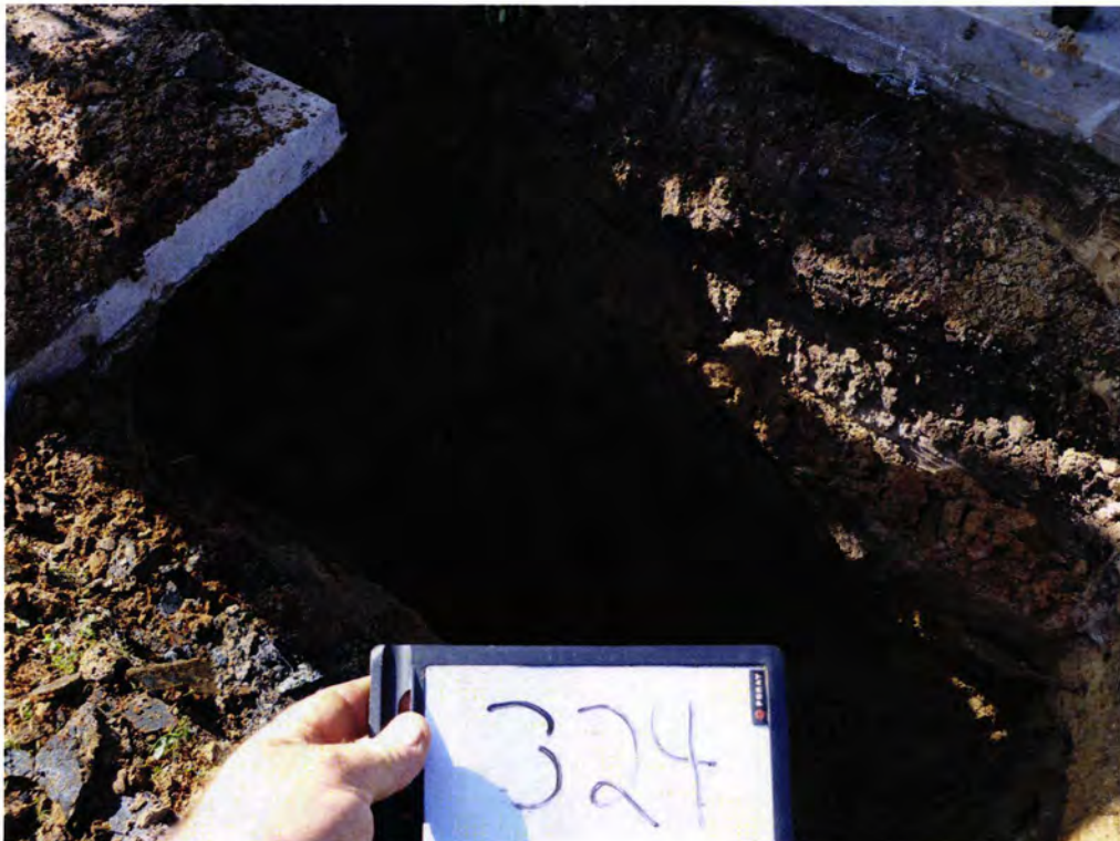
Picture 2: UST 324Ash tank pit.
